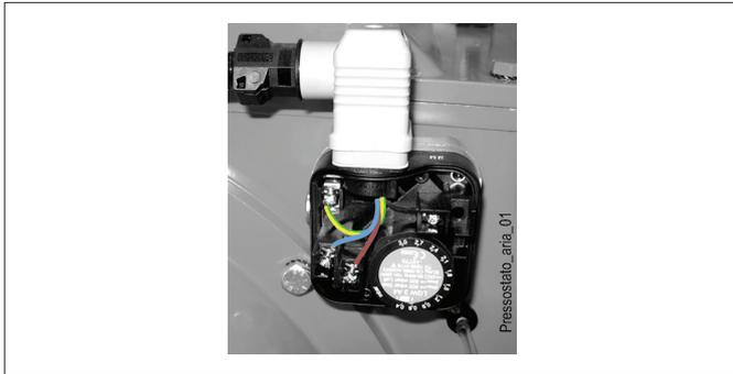
The gas pressure control switches (minimum and maximum) prevent the burner from operating when gas pressure does not lie between the expected range.
